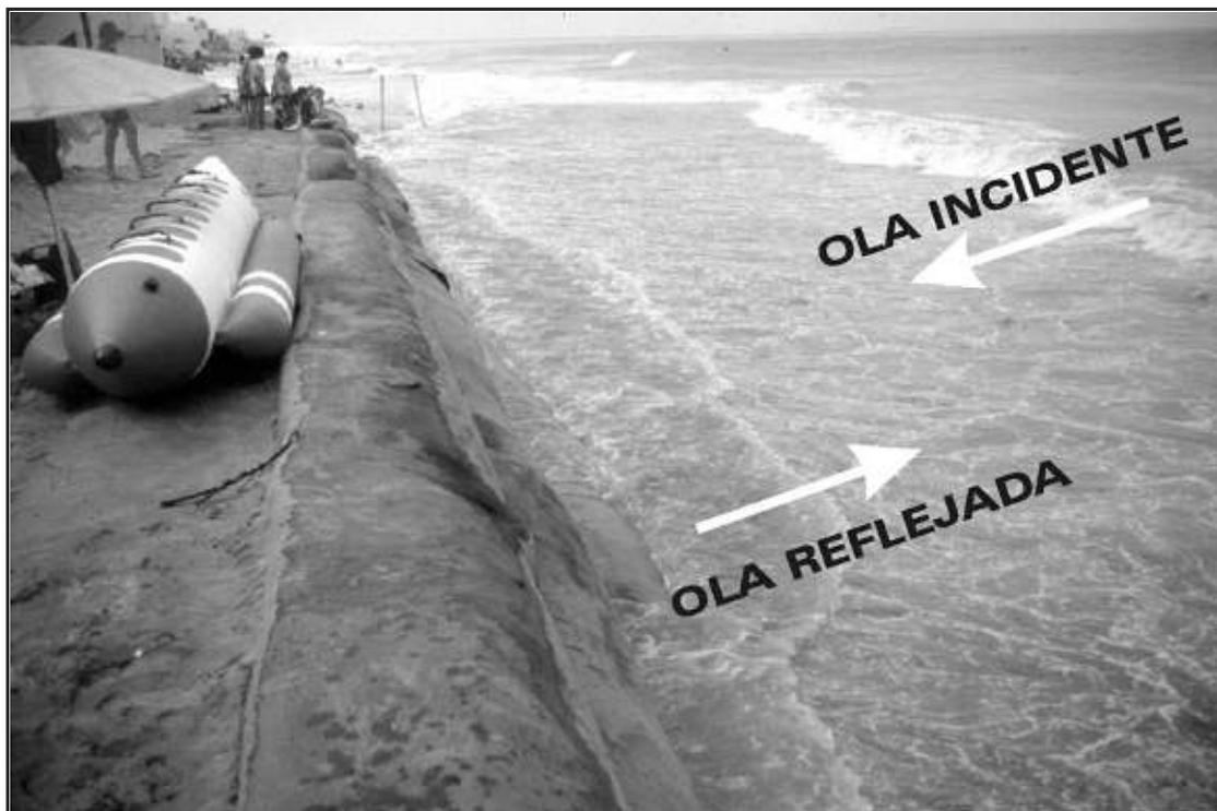
**FIGURA 7. DETERIORO DE LAS ESTRUCTURAS DE GEOTEXTIL.**
